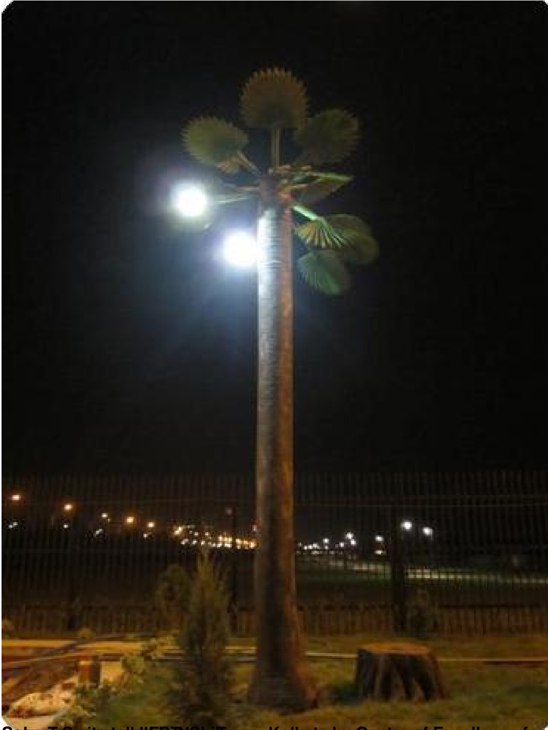
Solar Street Light LED Lamp, Newipun, Kolkata by Centre of Excellence for Green Energy and
