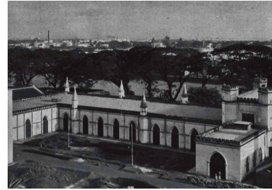
Old Building of Bengal Engineering College (1920)
