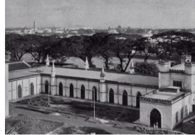
Old Building of Bengal Engineering College (1920)
